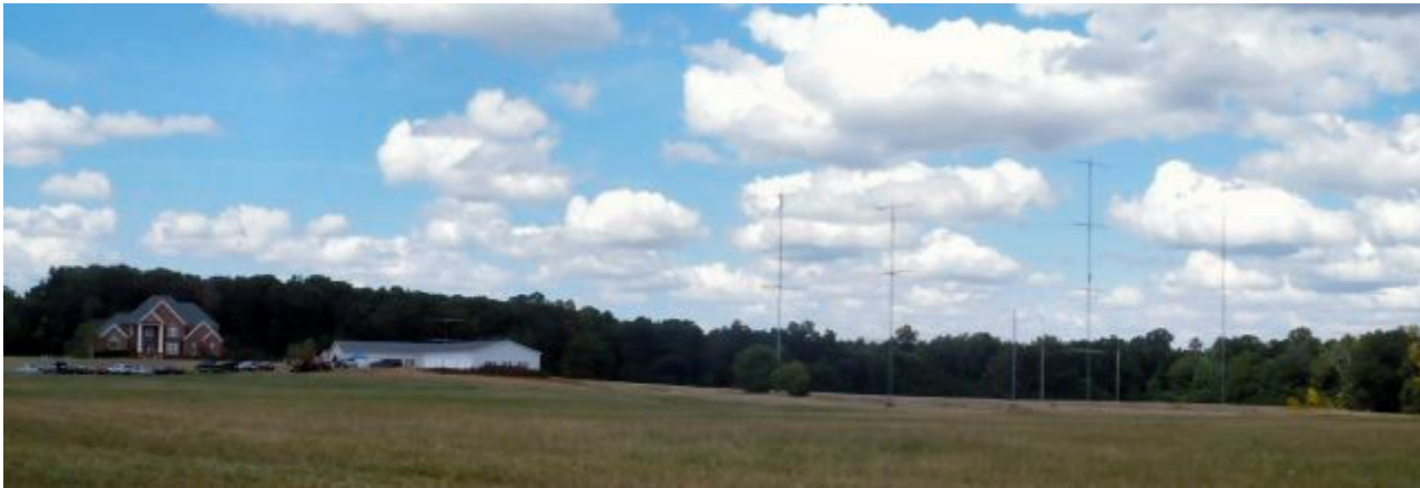
Just a few more antennas than the W4PM antenna farm!
